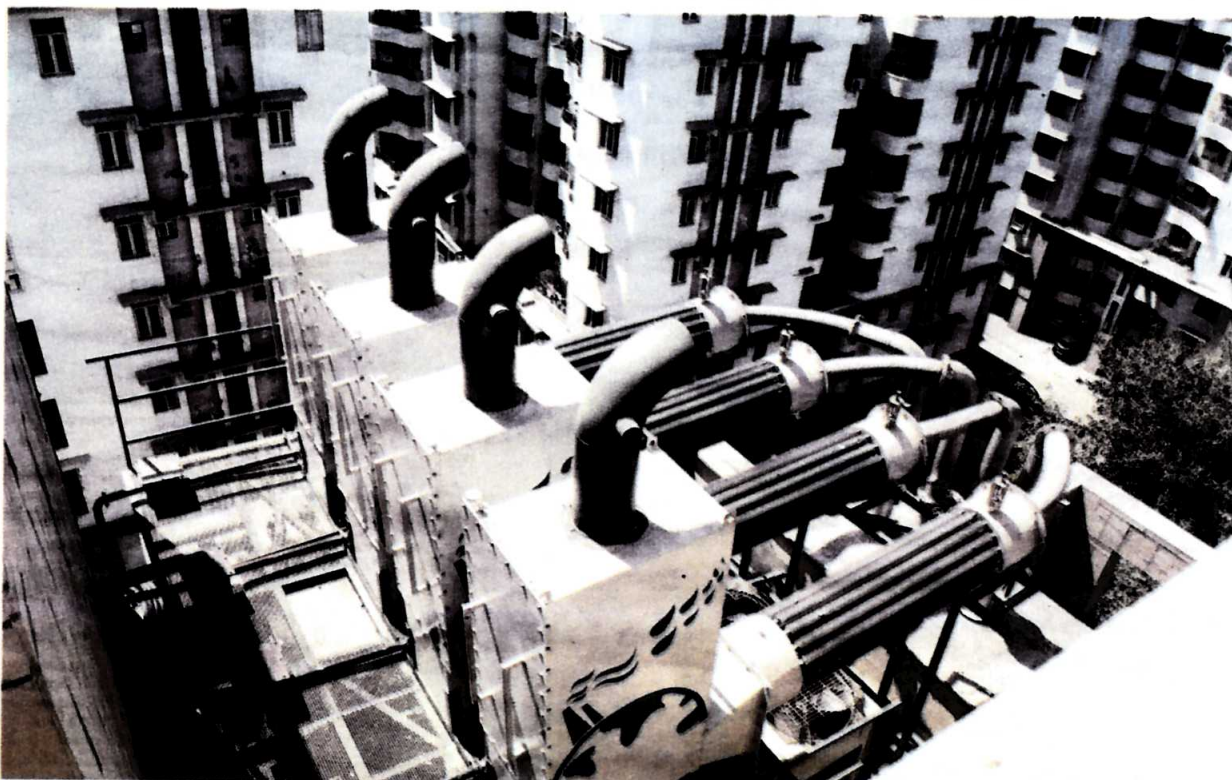
A device created by Chakr Innovation removes soot from the diesel general exhaust, to clean the air and allow ink to be created from soot, on a building in Gurgaon, a satellite city of New Delhi, India. — Picture by Reuters
